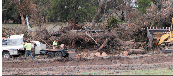
Contractors clear vegetation from the 20 acre site last week. The land has been approved for 110 dwellings, marketed as 'Heritage Bay' estate. G041616
